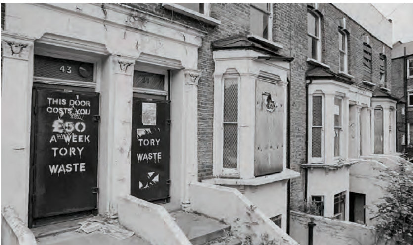
Image 4. Boarded-up houses on Waltherton Avenue, W9. (Photograph: Philip Wolmuth)
